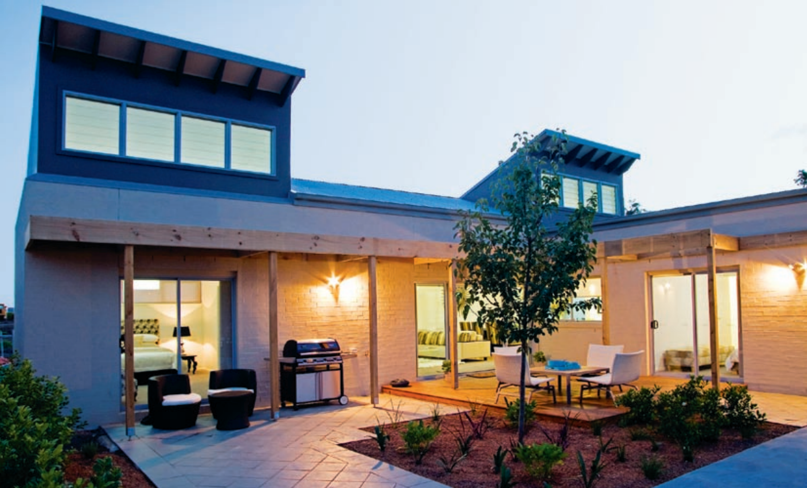
The Arbour, Berry NSW Construction by Masterton Constructions
